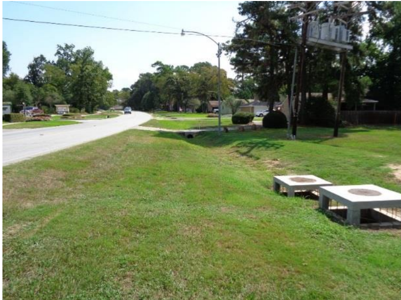
Improved inlets on Walden Road at GSU Easement
