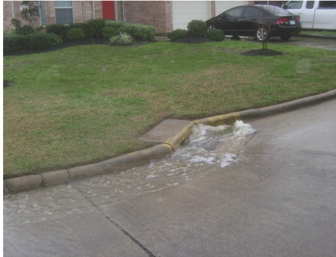
Angled inlets bypassing flow during short, hard rain event
