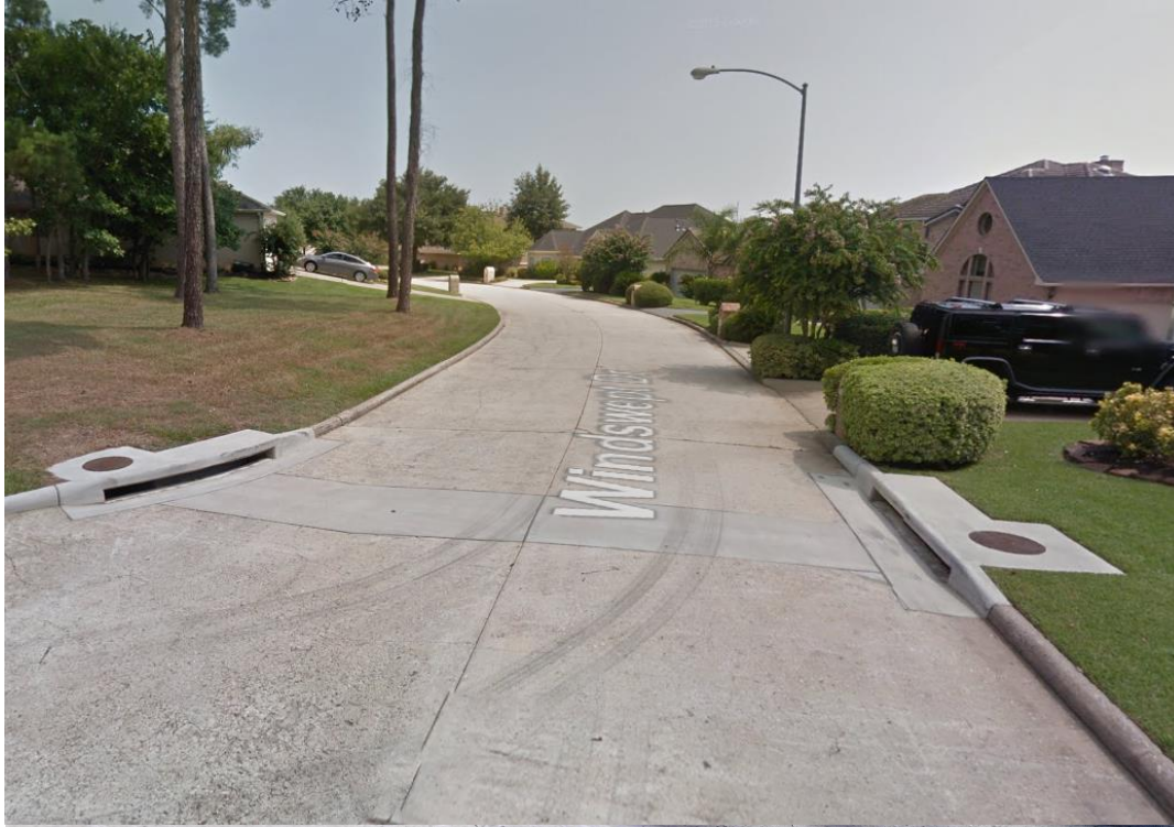
Installed 2 inlets at Vail Drive
