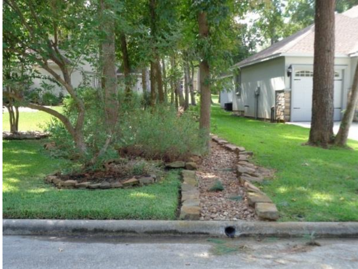
Existing Rock Drainage Swale constructed by property owner
