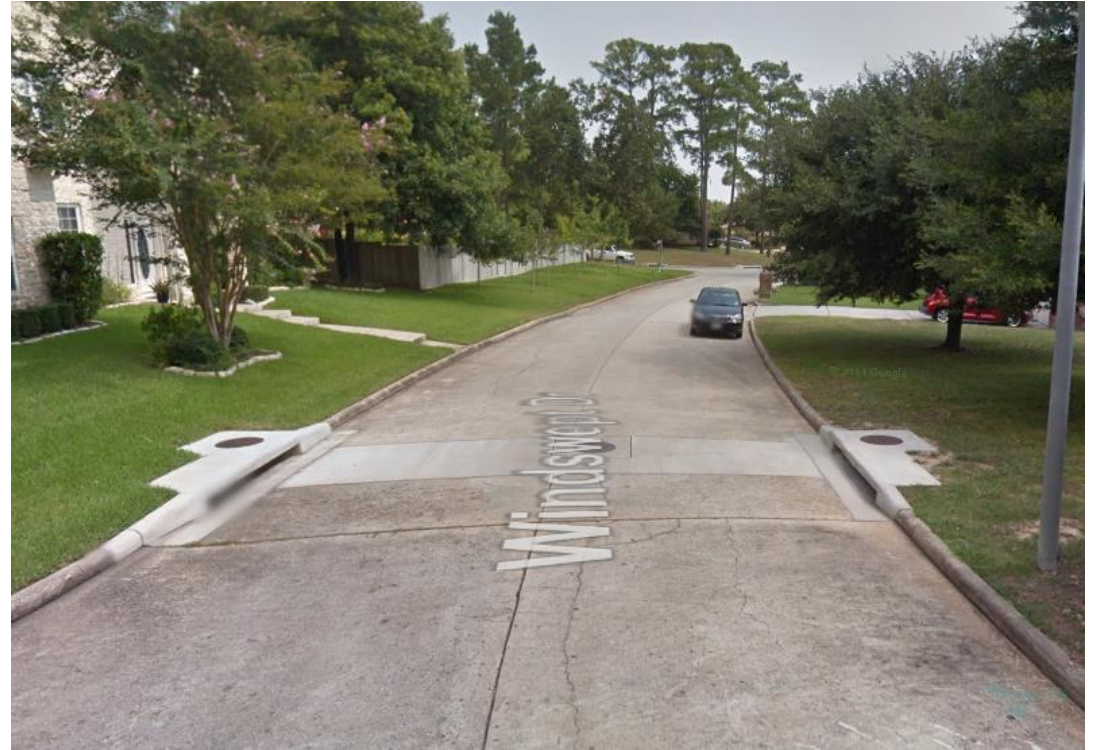
Installed 2 inlets at Sun Valley Drive
