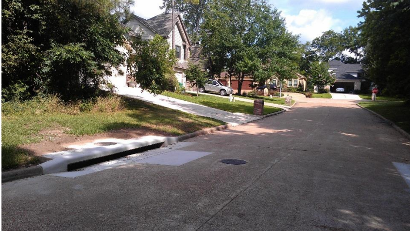
Upsized curb inlets and swale
